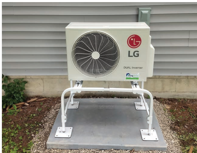
Cold-climate heat pumps must be elevated above the average maximum snow depth. Be sure to allow for free drainage below the unit.
